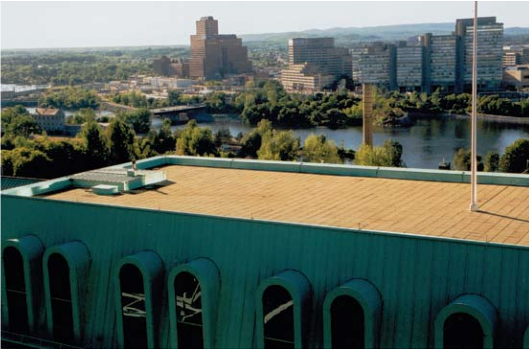
Figure 2. While acting as a ballast for waterproof roof membranes, light colored precast concrete paving slabs and concrete pavers also can reduce building energy costs and reflect damaging sunlight.
