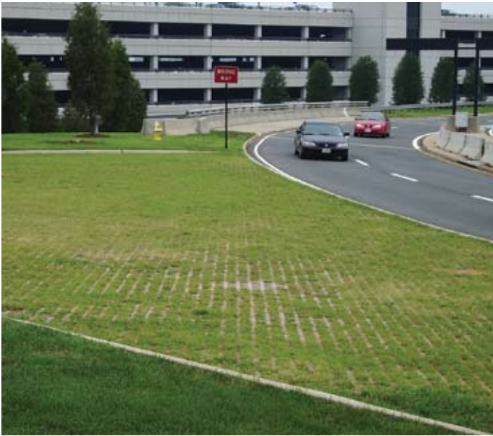
Figure 1. Concrete grid pavements are one way to introduce a cooler microclimate, help reduce the urban heat island and earn LEED® points.
